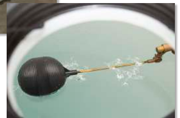
250-gallon holding tank, with brass float valve and supply plumbing
